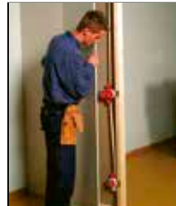
Mount the plaster-board/panelen.
