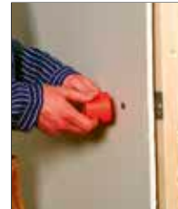
Search for the insert using HOLE IN ONE seeker 8:21 or Super-seeker 2000 and mark out the center.
