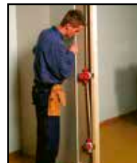
Monter gipsplate /panel.
