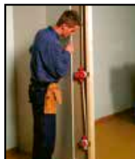
Monter gipsplate /panel.
